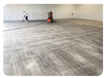
Monica vacuums and patches cracks to prepare for the Kopps' threelayer flooring system, which was applied over three consecutive mornings.
